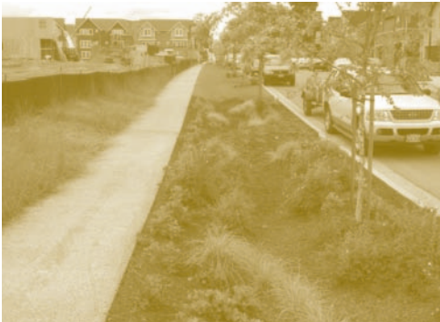
BIORETENTION AND PERVIOUS PAVEMENT ARE USED TO TREAT AND REDUCE RUNOFF
